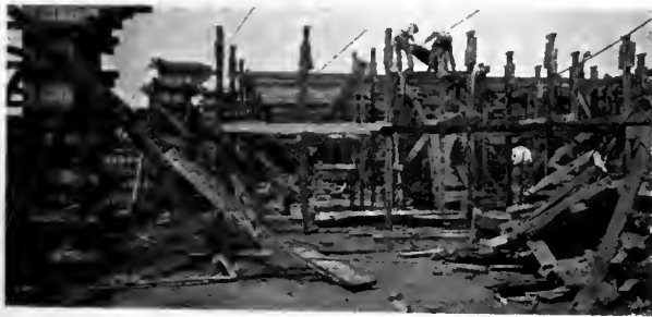
FIG. 2. SHOWING METHOD OF ERECTING SUPPORTS
